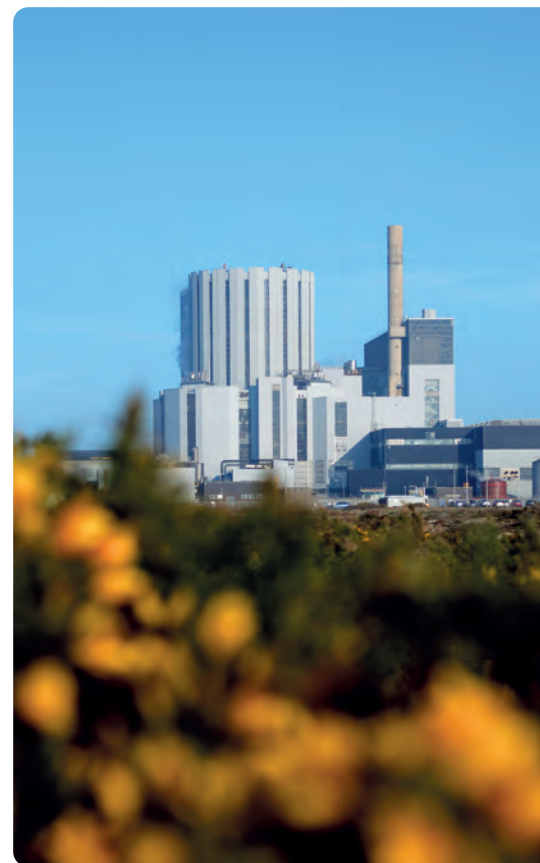
Dungeness B Nuclear Power Station
