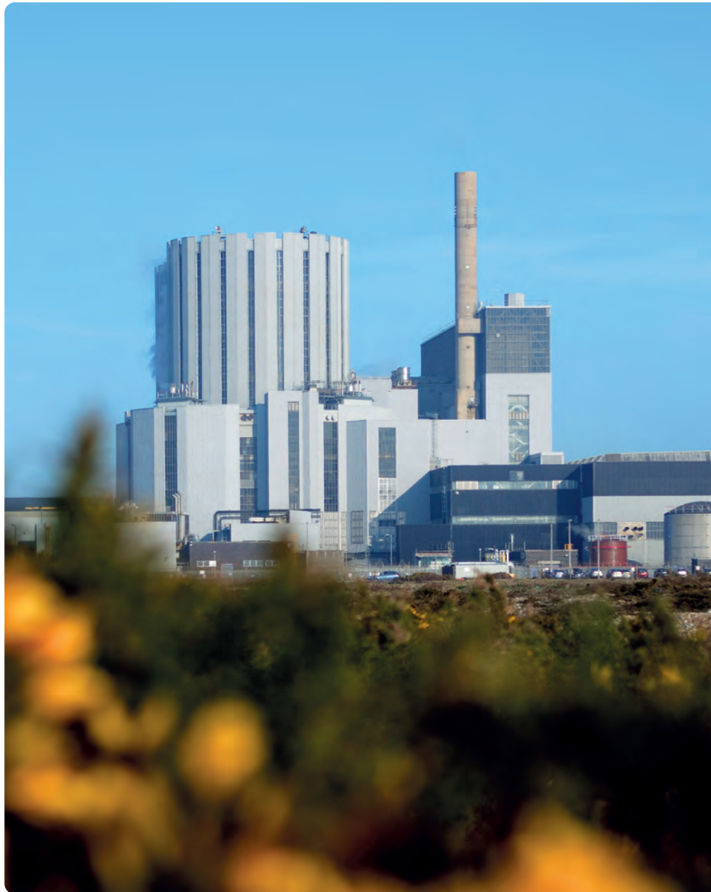
Dungeness B Nuclear Power Station
